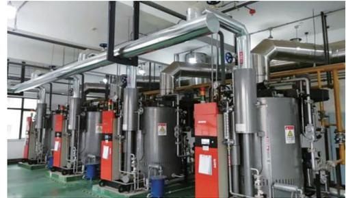
Low-nitrogen burners used for the gas-fired boilers in Beijing plant
