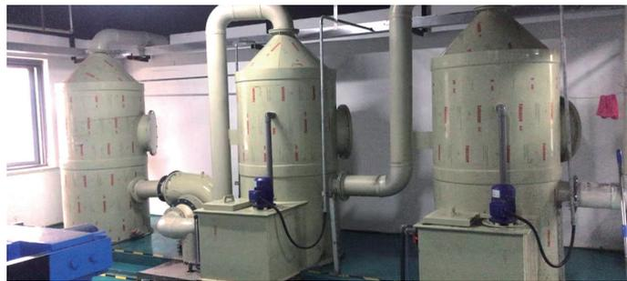
Harmless treatment of exhaust gases used for the sewage treatment system in Beijing plant
