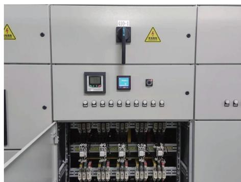
Reactive compensation technology for power grid system
