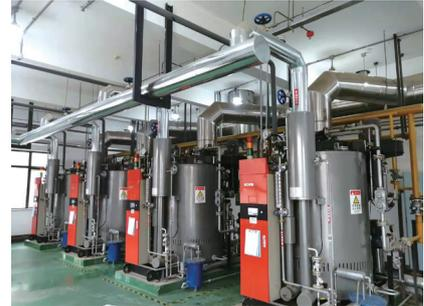
Low-nitrogen burners used for the gas-fired boilers in Beijing plant
